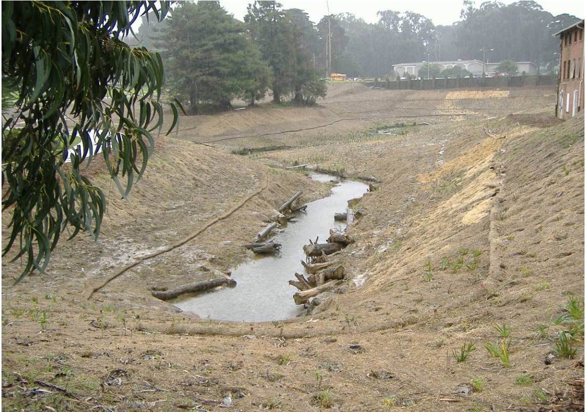
Figure 26: Completion of earthwork and grading activities. Looking south.
