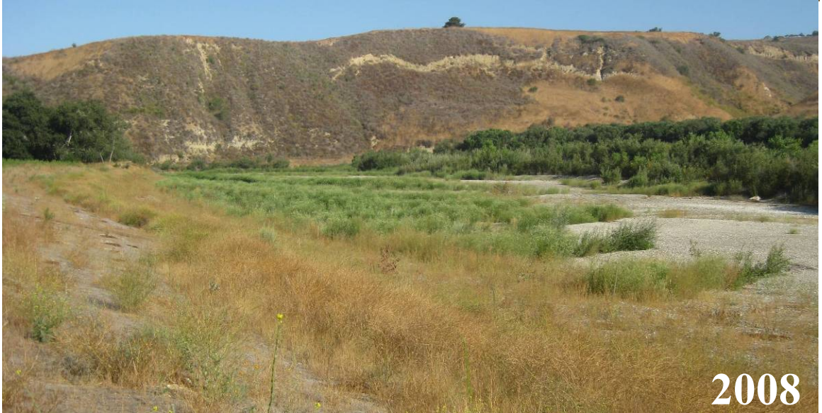
Figure 52: Photos showing pre- (2006), as-built (2007), and 1 year post-project (2008) views of the project.
