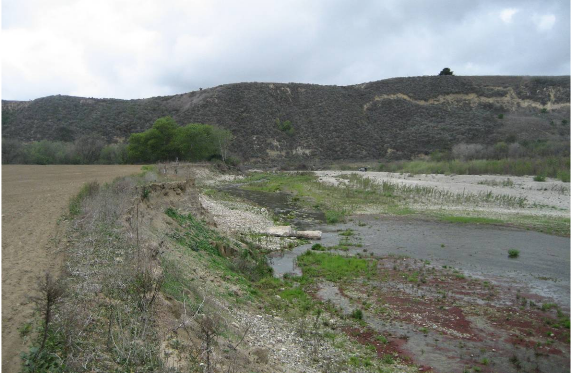
Figure 40: Pre-project view of project site looking downstream.
