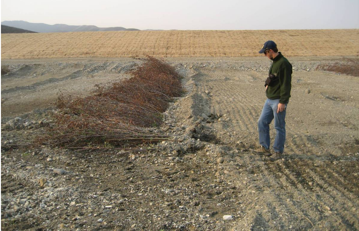
Figure 47: View of a completed willow baffle.
