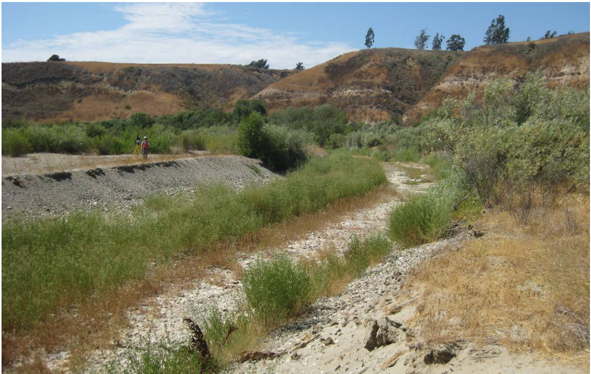
Figure 56: The bypass channel experienced significant bank erosion and vegetation growth.
