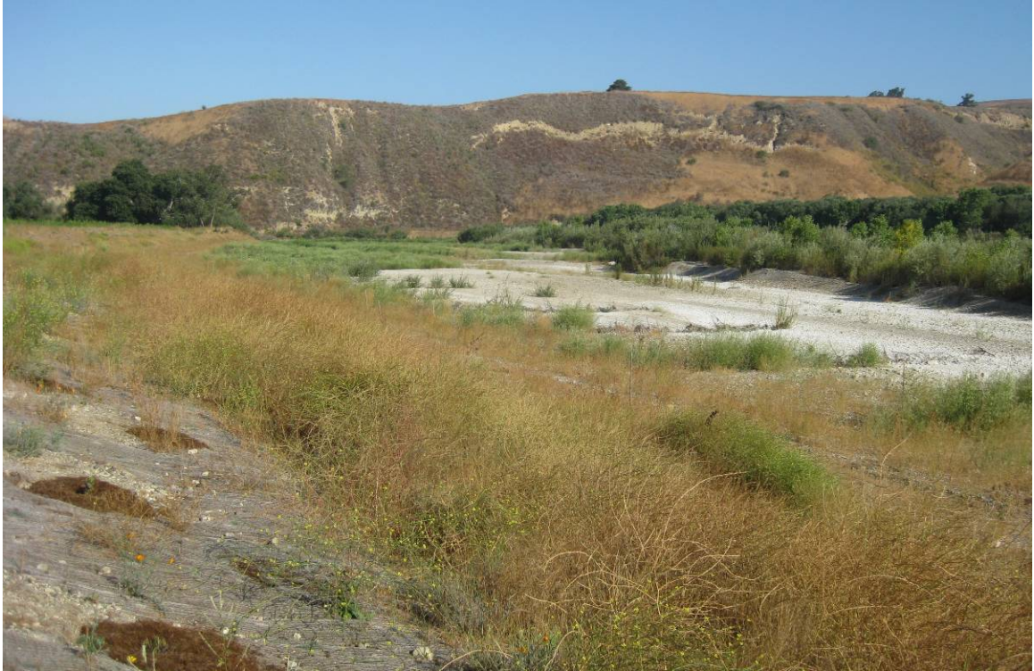
Figure 55: The planted vegetation is becoming established. The willows in the willow baffles (green) are taking shape.
