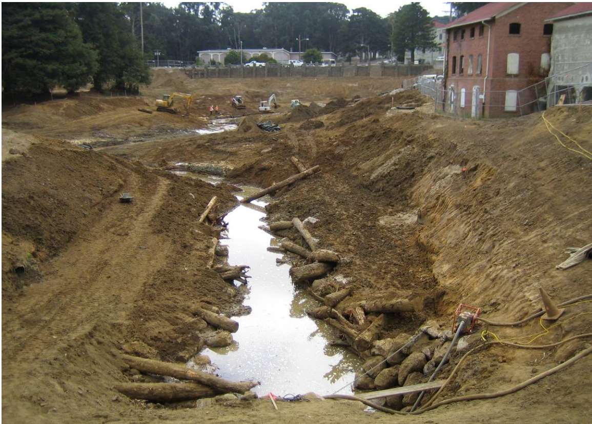
Figure 25: Large woody debris used to aid in bank stabilization.
