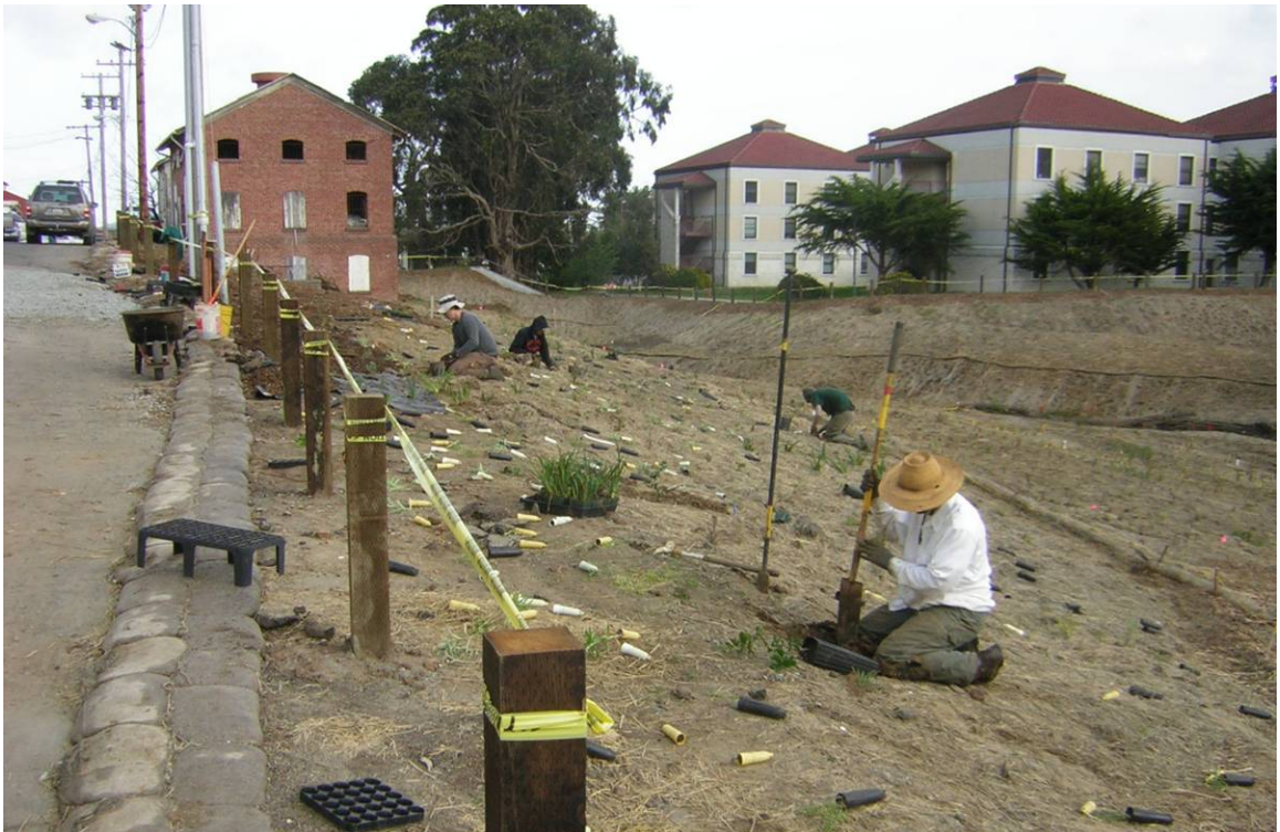
Figure 27: Planting riparian vegetation was the final aspect of construction.
