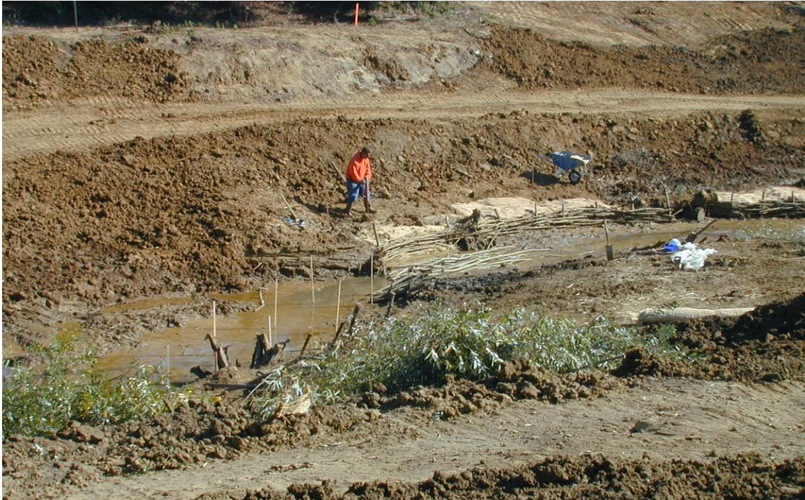
Figure 24: Installation of woven willow walls for erosion protection at meander bends.
