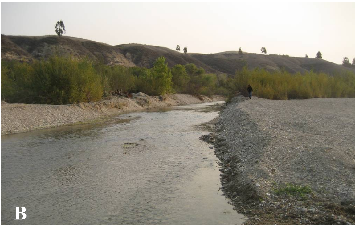
Figure 46: The downstream end (location B) of the temporary construction bypass channel.
