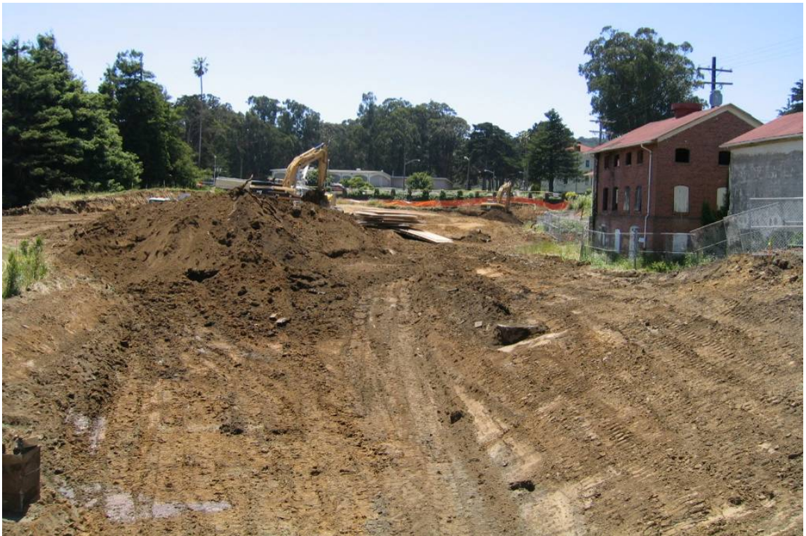
Figure 19: Removal of contaminated soil with an excavator (looking south).
