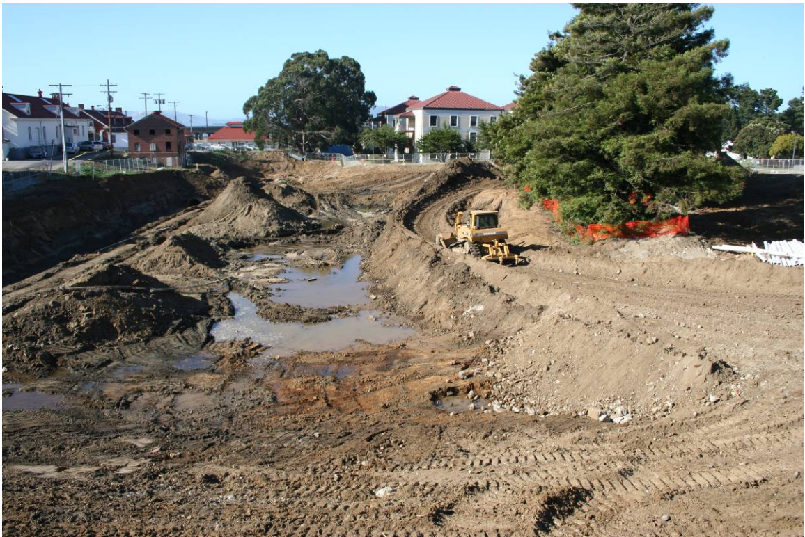
Figure 21: Groundwater encountered during excavation of onsite soils.
