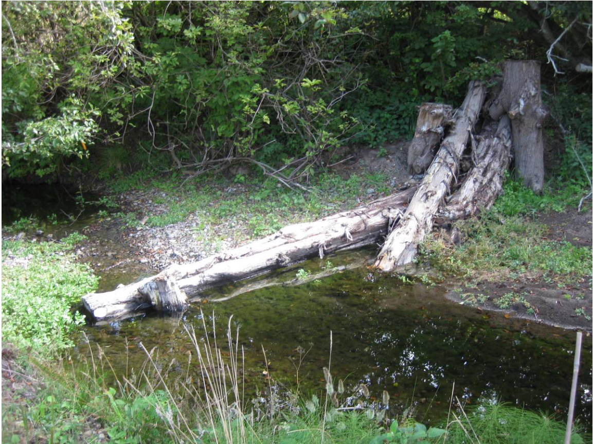
Figure 13: Use of demolition materials to construct grade stabilization and to increase in-stream habitat channel complexity (Redwood Creek, Marin County).
